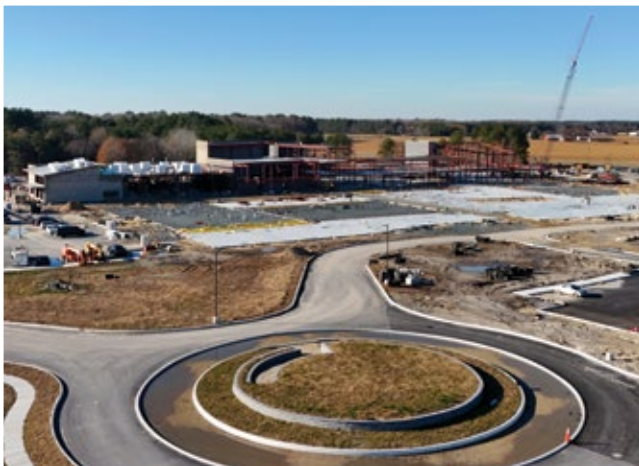
SUSSEX COUNTY VOCATIONAL TECHNICAL SCHOOL CONSTRUCTION
